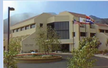
Twenty million dollars worth of roofs, exterior walls and below grade waterproofing went into Pepperdine University's Malibu campus.
